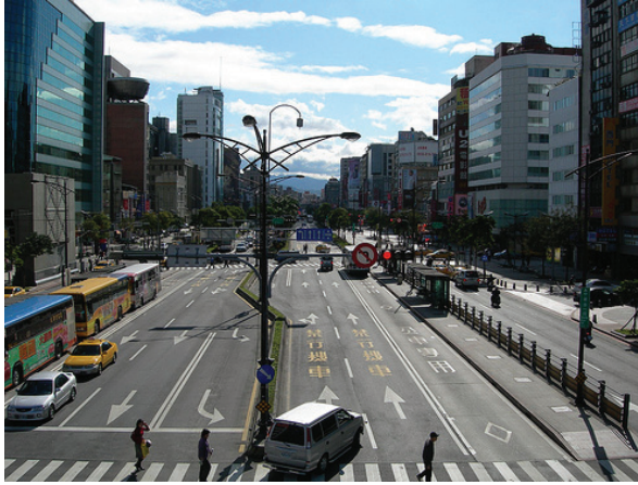
Fig. 10. Typical Taipei City bus lanes.
